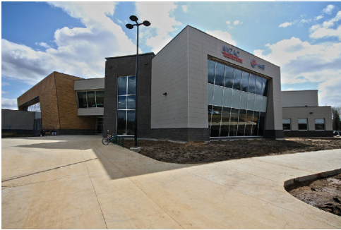
Anzac Community Recreation Centre
