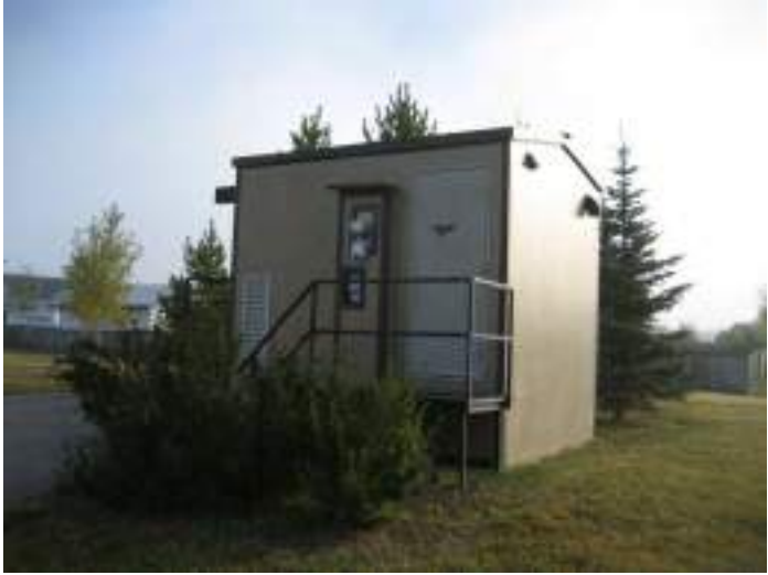
Photo 1: Pump house, showing elevated floor
