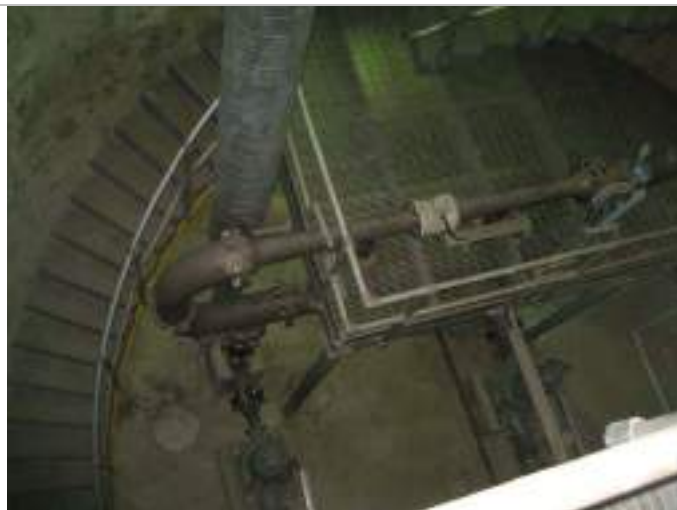
Photo 2: Pumps and discharge piping
