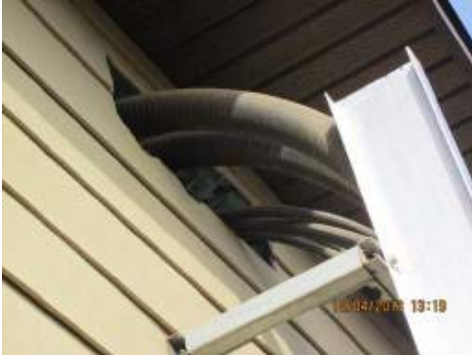
Photo 9: Install cover or seal siding where electrical cables enter at southeast corner.
