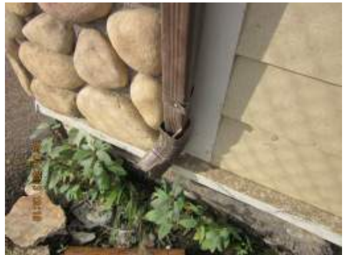
Photo 8: Repair and extend downspout at southeast corner.
