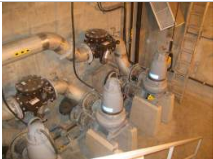
Photo 1: Dry well – Pumps, discharge valves and piping.
