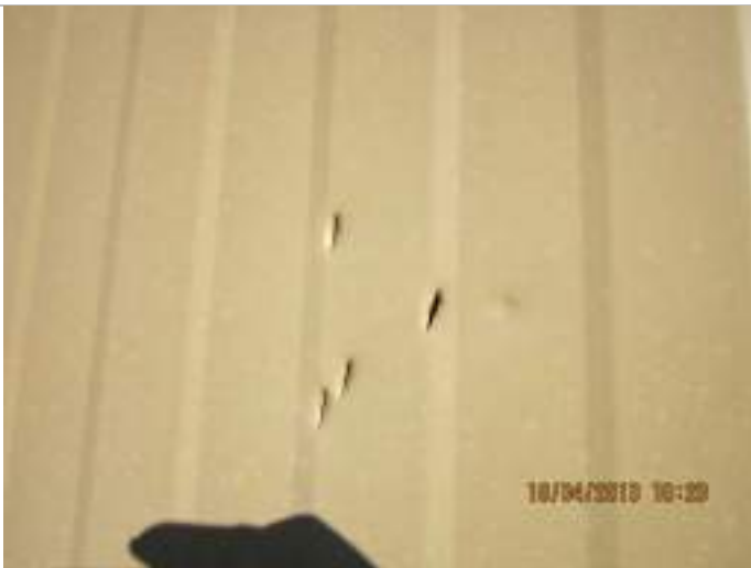
Photo 1: South Exterior Wall with damage to cladding.
