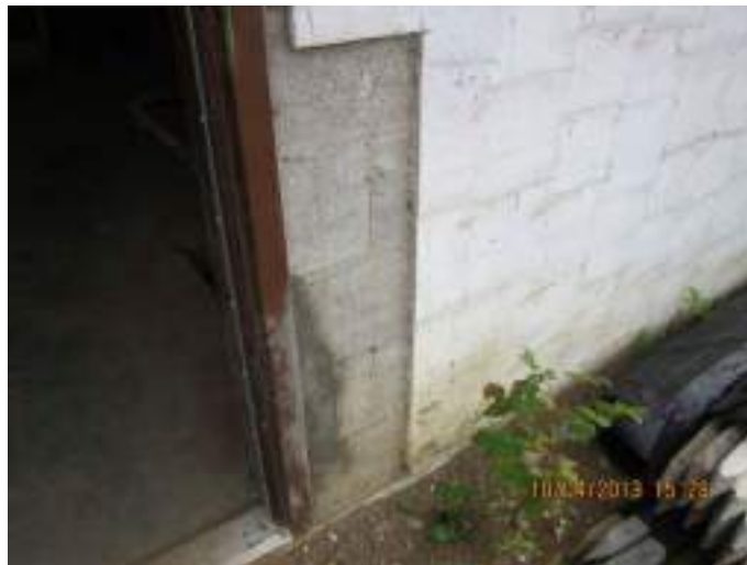
Photo 14: Parging has been removed on the outside wall near the door to the Dry Well.
