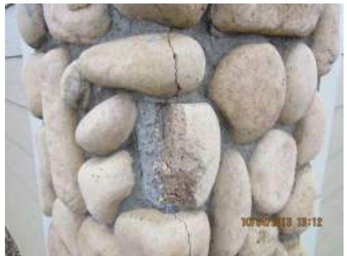
Photo 4: Crack in stone and mortar on northeast corner.
