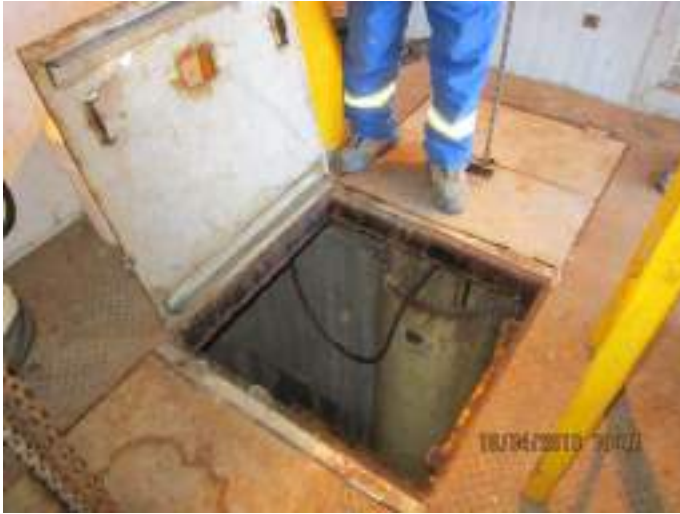
Photo 9: Wet Well access hatch. Utilize fall protection system to access Wet Well.
