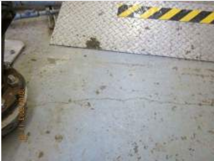
Photo 5: Paint is peeling off of main floor concrete slab.
