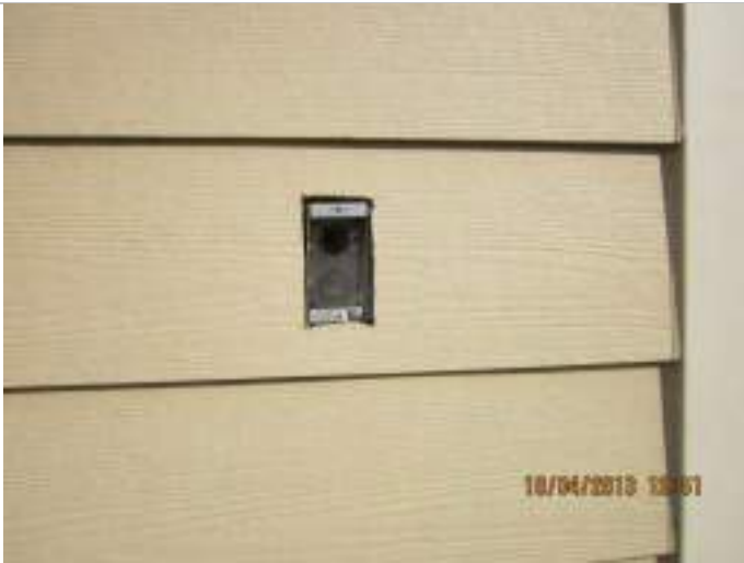
Photo 1: Exposed electrical outlet box on outside wall.
