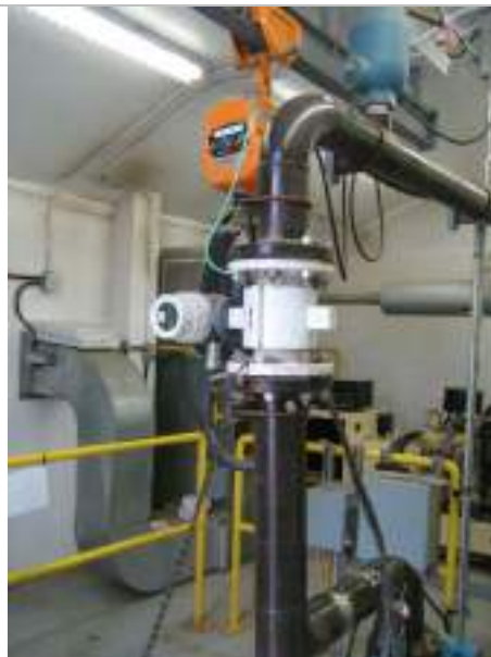
Photo 2: Discharge piping, flow meter.
