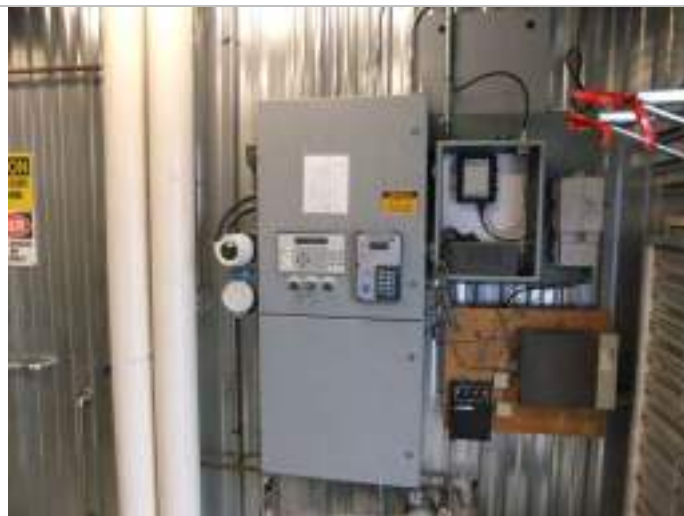
Photo 2: XBT Magelis controller (obsolete and broken buttons) and communication panel without door.
