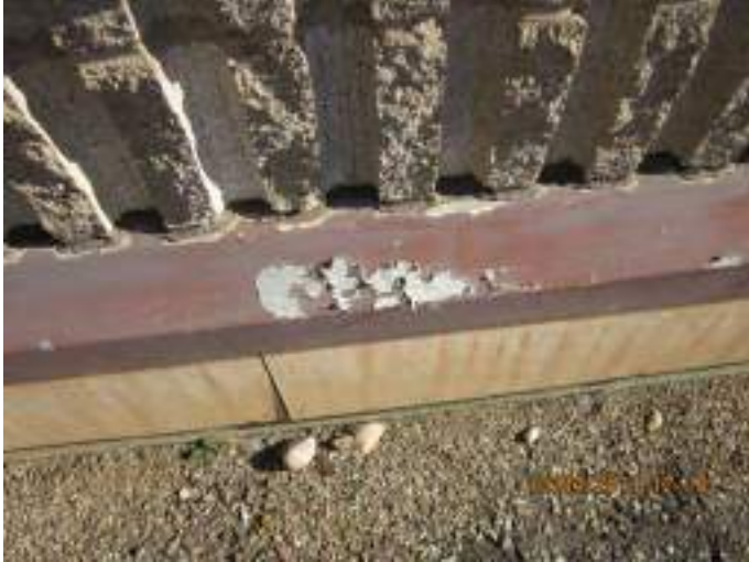
Photo 5: Paint peeling off metal wall flashing.
