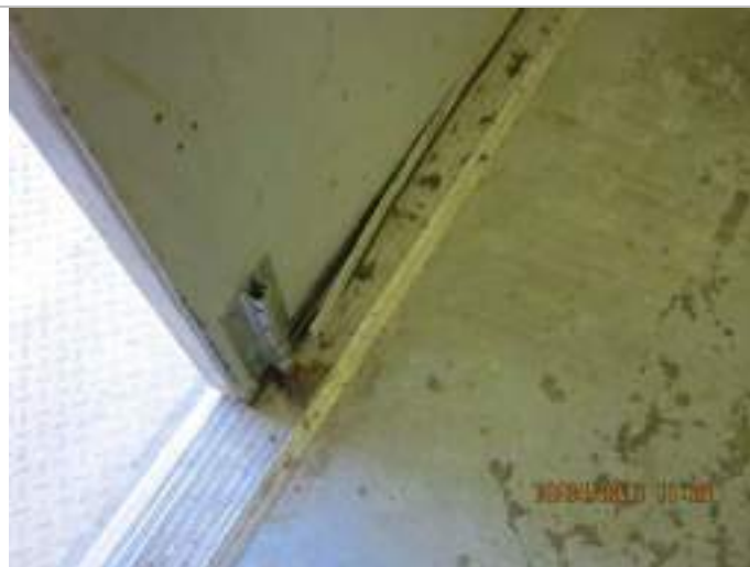
Photo 10: Bent molding on the inside of the door at the bottom.
