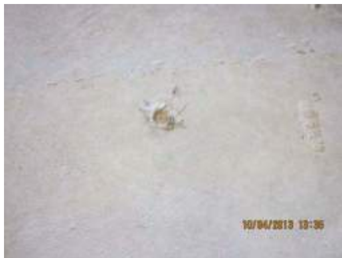
Photo 14: Bolt cut off and exposed in the Dry Well main floor concrete slab.
