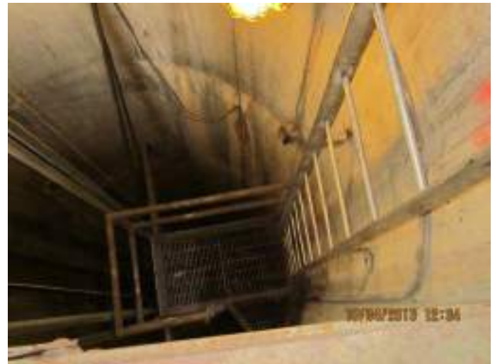
Photo 12: Access ladder to Wet Well. Use fall protection system when using ladder.
