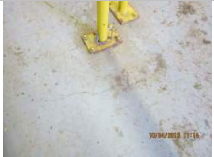
Photo 6: Crack in main floor concrete floor slab.
