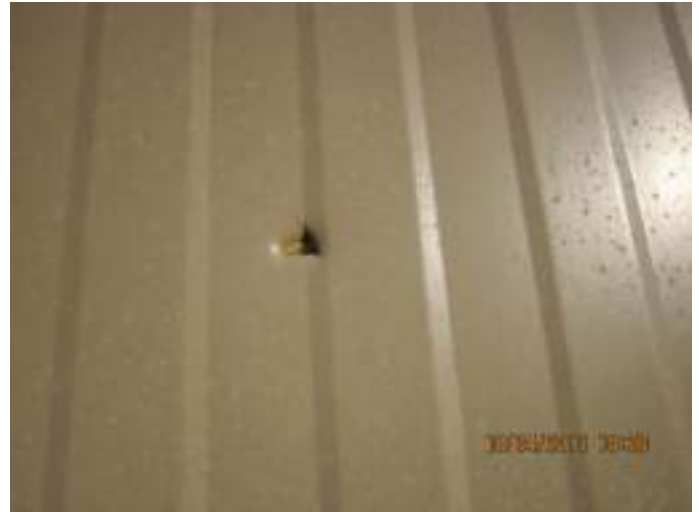
Photo 2: Perforation in cladding.
