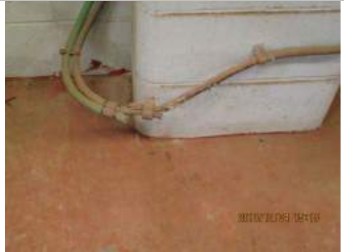
480 and 600 VAC ground systems seem to be connected together. No site ground was found.
