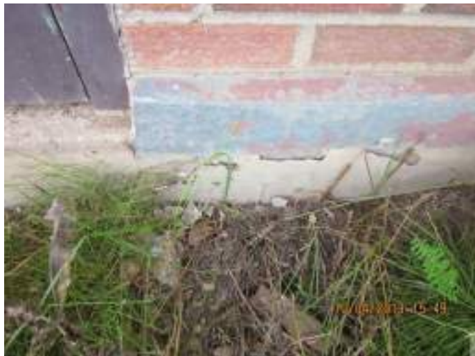
Photo 13: The concrete foundation is spalling on the north side near the double doors.
