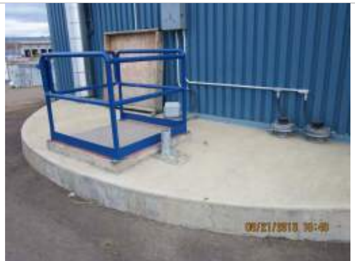
Photo 10: Rust staining on the antennae foundation.
