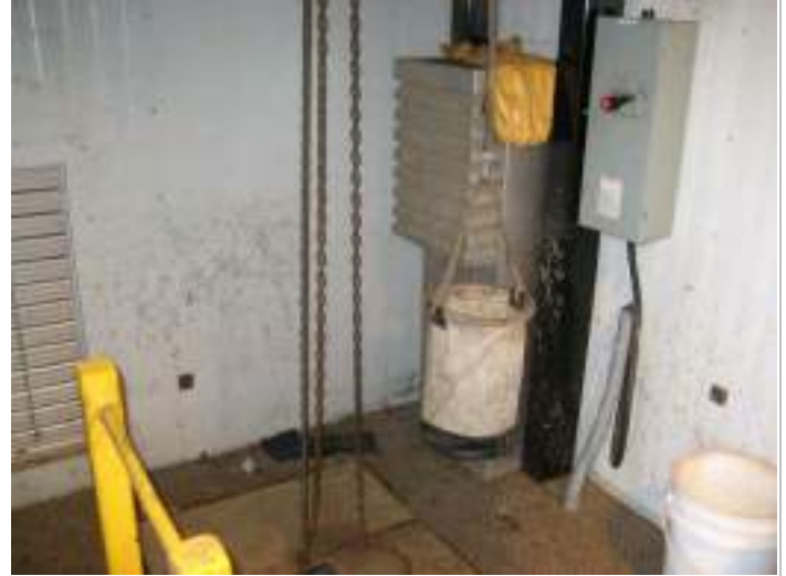
Photo 2: Wet well access hatches, including heater and ductwork.
