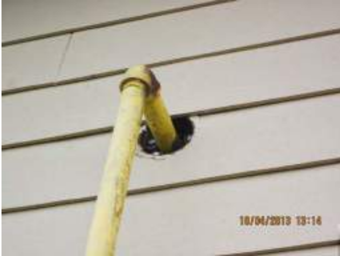
Photo 5: Caulk siding around gas line.
