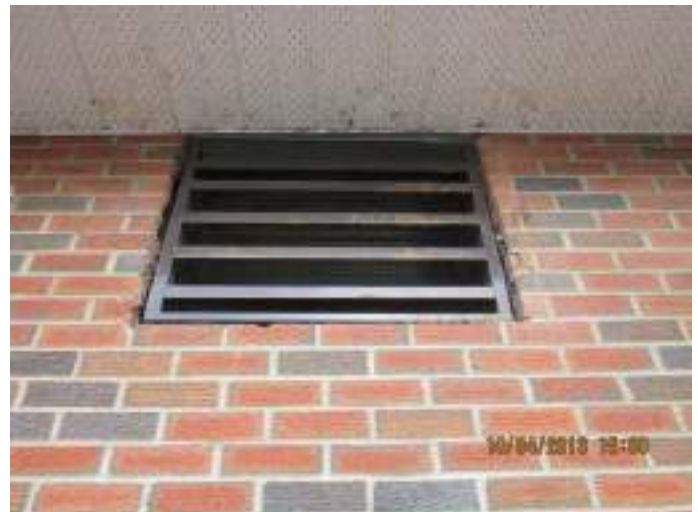
Photo 4: Caulk the gap between the louver and the brick near the entrance to the Wet Well.
