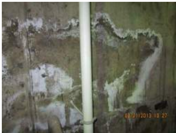
Photo 2: Water staining on Dry Well south wall.
