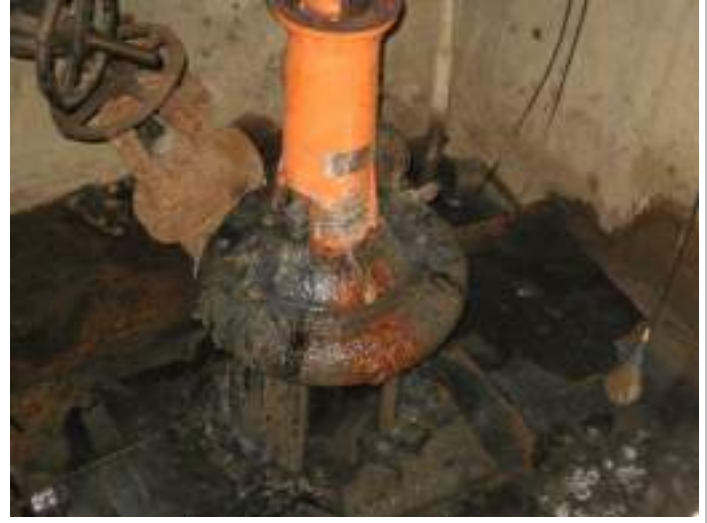
Photo 2: Pump #1 – Leaking seals.
