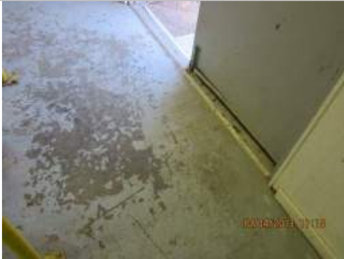
Photo 5: Paint is peeling off of main floor concrete slab.
