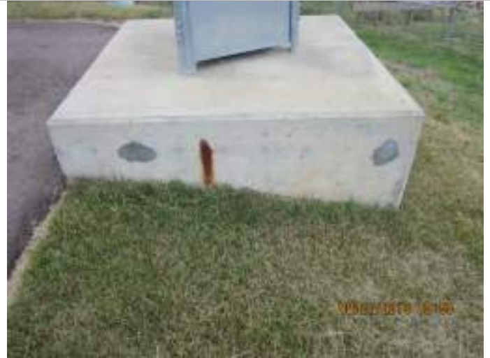
Photo 10: Rust staining on the antennae foundation.
