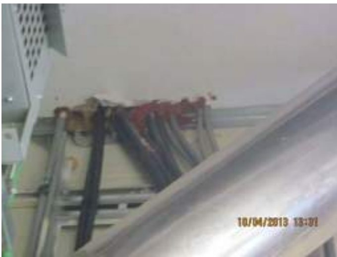
Photo 11: Repair ceiling and re-caulk where electrical cables enter ceiling.
