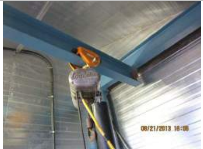
Photo 10: Monorail and crane on the Wet Well side of the Station.
