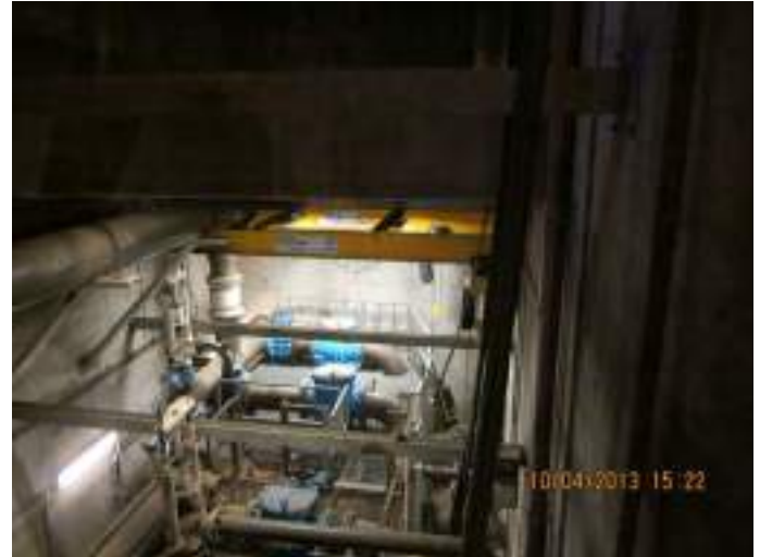
Photo 10: Monorail cranes SN 1250-3 and SN 1250-4 at the bottom of the Dry Well. The crane inspection certificates may have expired.
