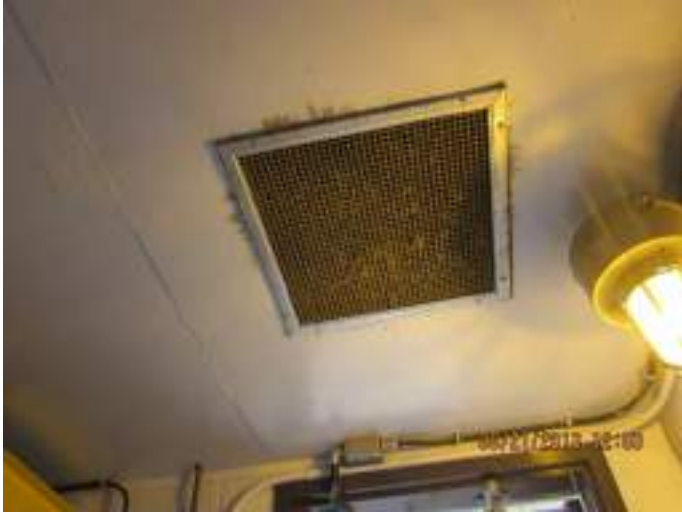
Photo 5: The Wet Well ceiling vent is clogging with dust and debris and requires cleaning.
