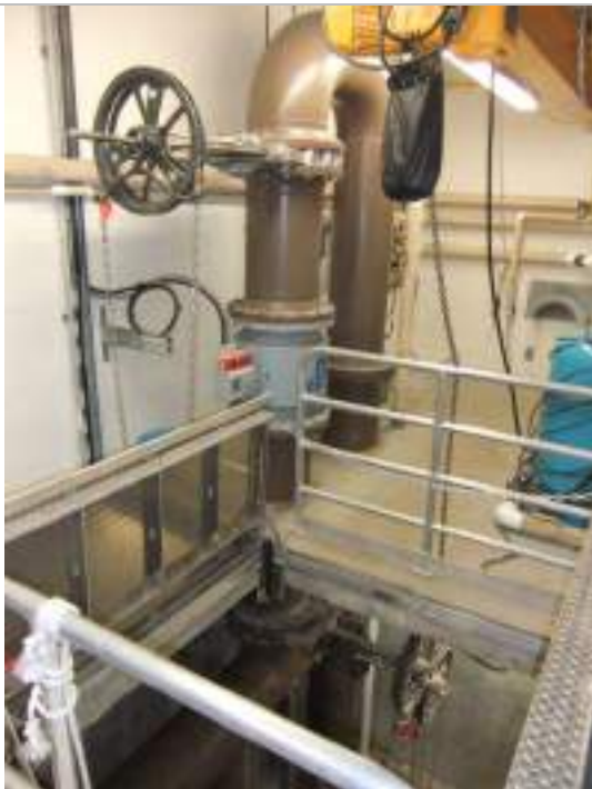
Photo 3: Upper and lower discharge piping.
