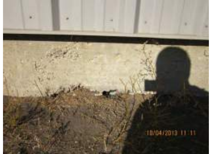
Photo 2: Voids and segregation in concrete foundation.
