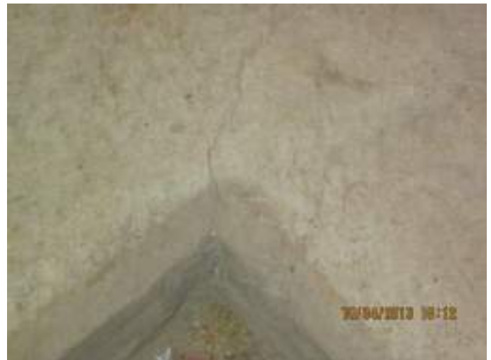
Photo 8: Shrinkage cracks in the MCC housekeeping pad on the Dry Well side.
