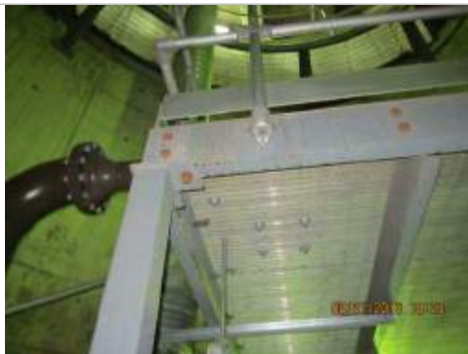
Photo 2: Water staining on Dry Well south wall.
