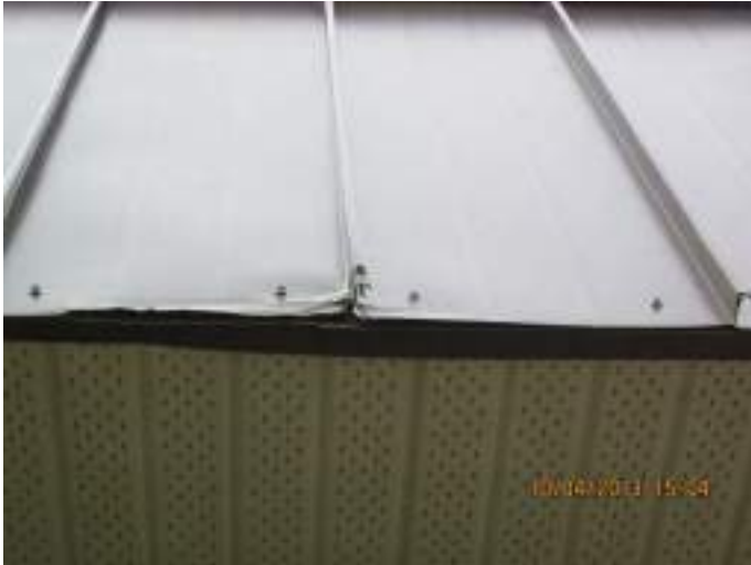
Photo 5: Repair the damaged metal siding on the north side.
