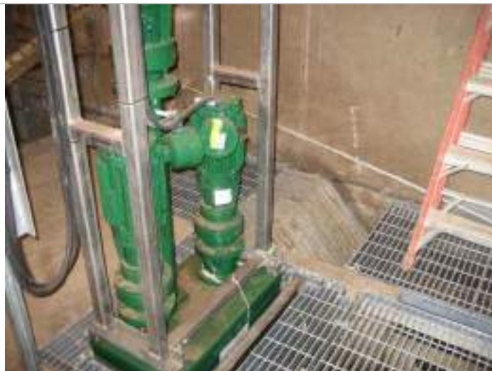
Photo 2: Grinder & bypass channel.
