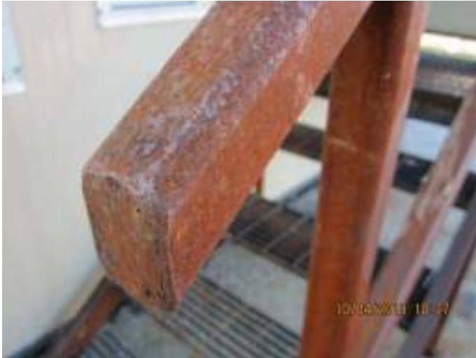
Photo 5: Corrosion on Wet Well outside stair handrail.
