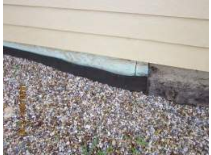
Photo 2: Exposed fiber board and insulation at building foundation.
