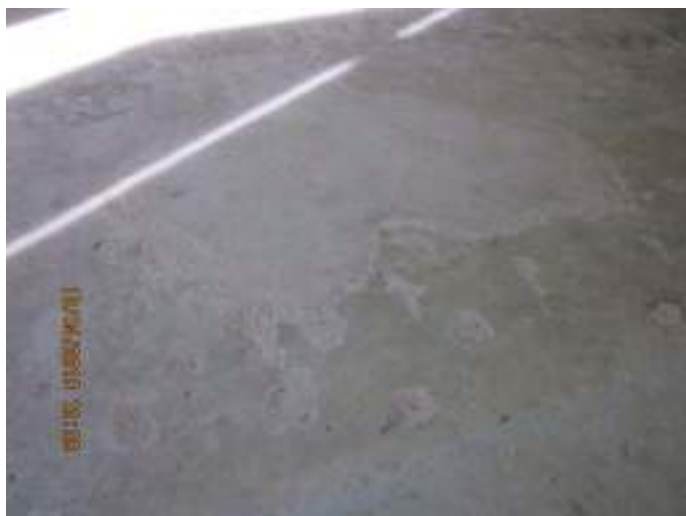
Photo 13: Patches in the Dry Well main floor concrete slab.
