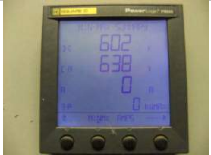
Photo 2: Current and power not indicating
