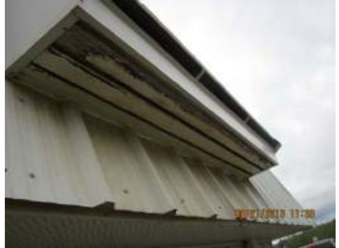
Photo 6: Paint is peeling off the underside of louver slats and requires sanding and re-painting.
