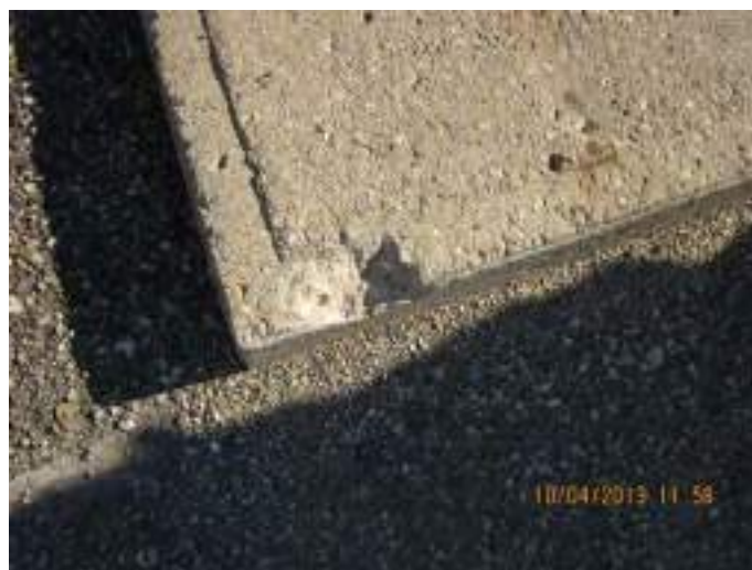
Photo 4: Spall in Dry well apron slab.
