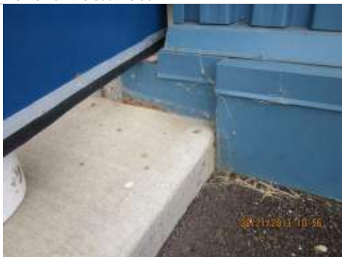
Photo 5: Missing section of metal siding on the bottom of the wall on the south side.
