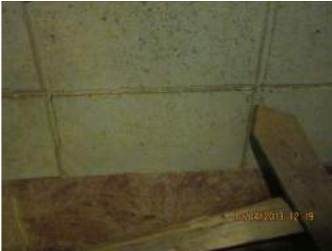
Photo 9: Cracks in joints of masonry block wall in Wet Well.
