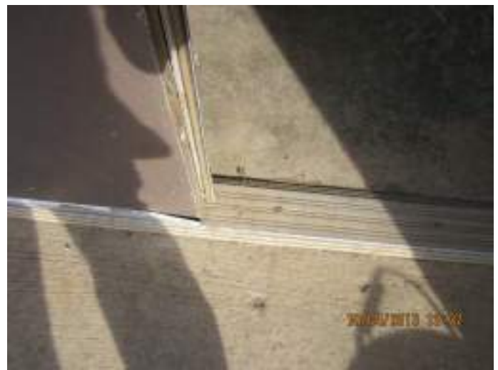
Photo 12: Fix bent door molding on Dry Well door.
