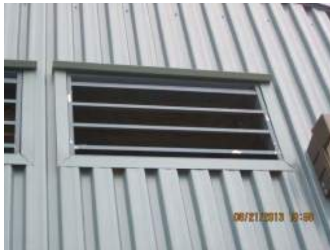
Photo 6: Loose chipped paint on the exterior wall louvers
