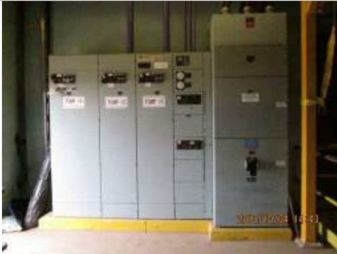
All 480VAC equipment seems to be approaching end of life.
