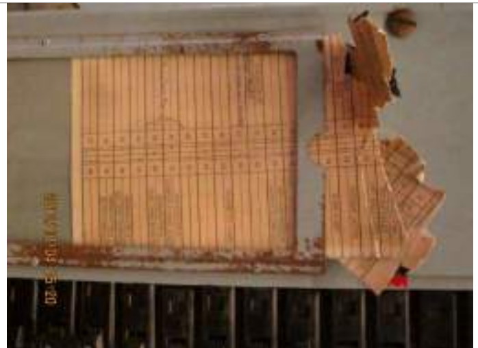
All panelboards supplies to be identified.
