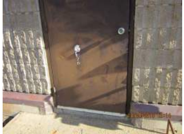
Photo 6: Paint peeling off Dry Well steel door.
