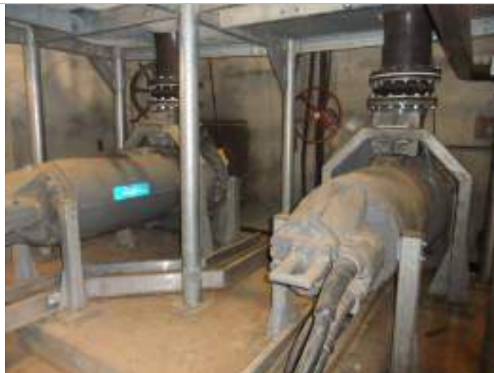
Photo 2: Two new pumps (P-003 & P-004) & piping.
