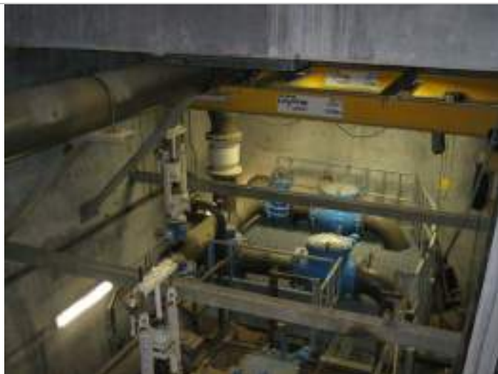
Photo 1: Dry well - discharge valves and piping.
