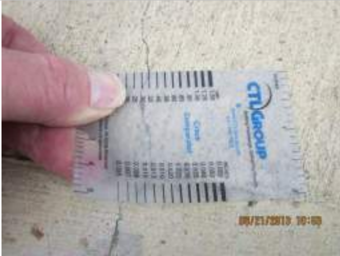
Photo 9: Cracks in the roof slab over the Wet Well greater than 0.3 mm.
