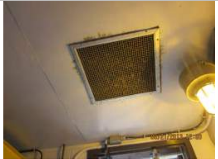
Photo 2: The pressure balancing is 'off' (notice dust trail along door and vent is fill with dust below).
