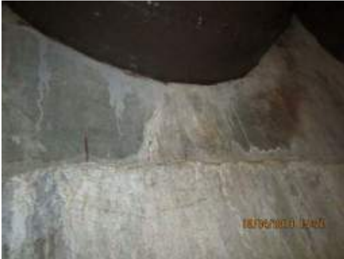
Photo 9: Shrinkage cracks in the Wet Well wall where a pipe passes through the wall.
