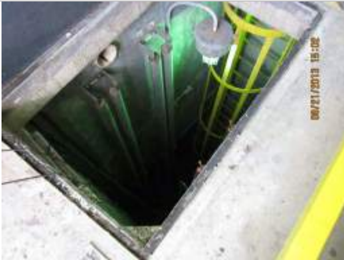
Photo 9: Wet Well access hatch, ladder, and safety cage.
