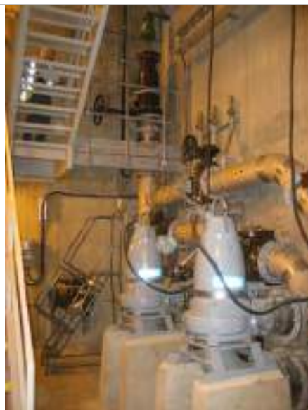
Photo 3: Discharge piping, including flow and pressure monitoring.
