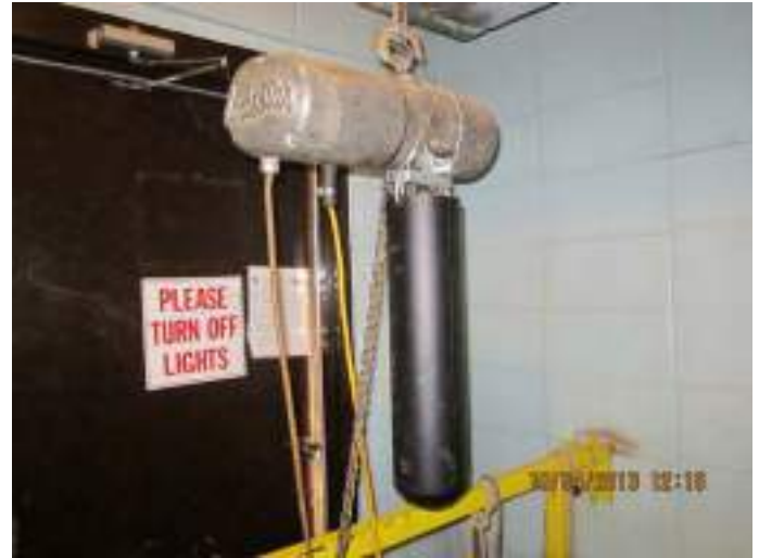
Photo 10: 1/2 ton monorail hoist in Wet Well. Monorail beam not labeled with safe working load.
