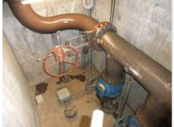
Photo 2: Dry well – discharge piping.
