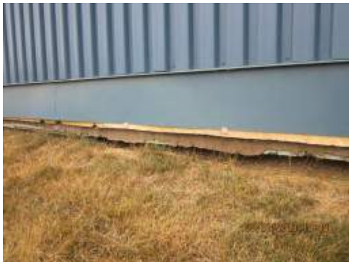
Photo 5: Missing section of metal siding on the bottom of the wall on the south side.
