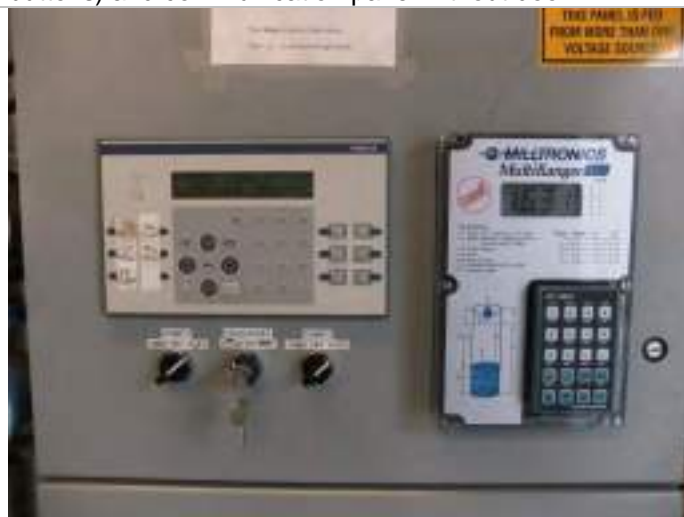
Photo 2: XBT Magelis controller (obsolete and broken buttons) and communication panel without door.
