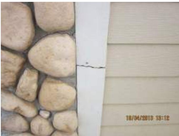
Photo 3: Crack in siding trim on northeast corner.
