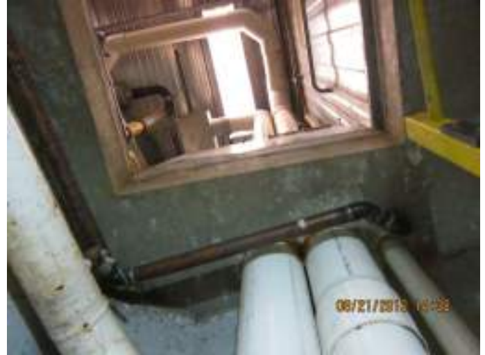
Photo 6: Accessing Dry Well Valve Pit is awkward with existing ladder and hand holds.
