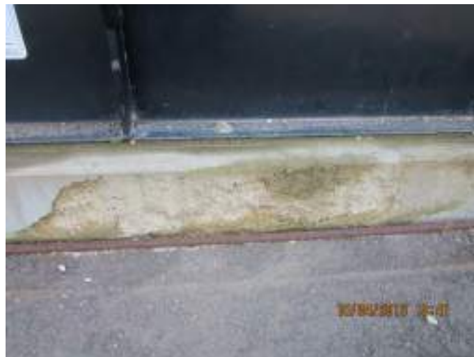
Photo 20: Generator concrete slab is spalling and needs repair.
