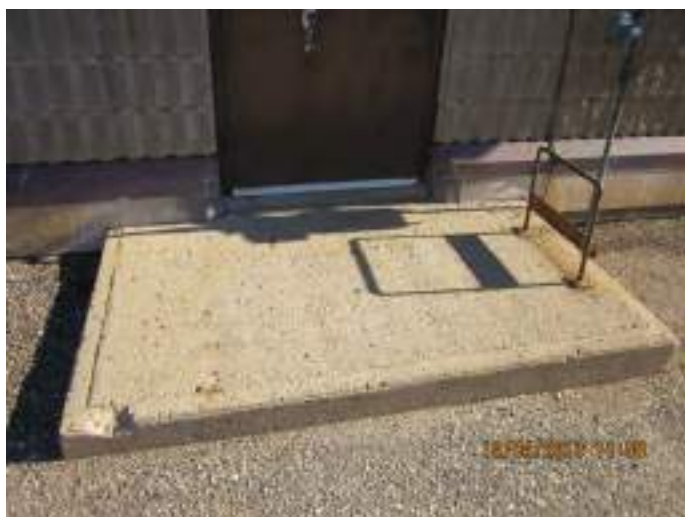
Photo 3: Dry Well apron slab.
