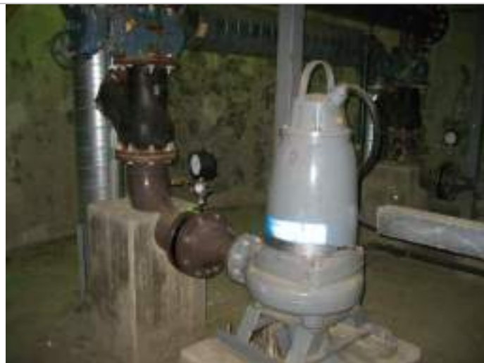
Photo 1: SWP – 401 & discharge valves, piping
