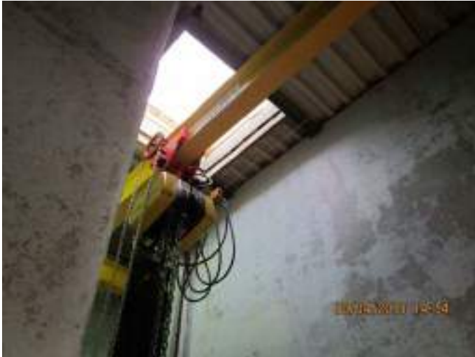
Photo 1: Monorail crane SN 1250-1 over the Wet Well. The rated capacity and inspection sticker are not visible.
