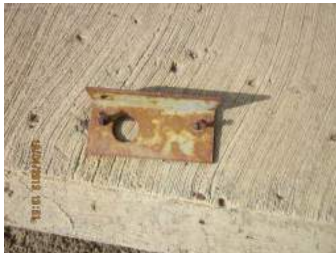
Photo 18: Door stop angle has corroded and is fastened to the apron slab with nails at Dry Well.
