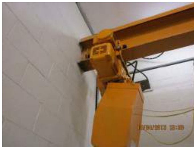
Photo 16: 2 tonne monorail on Wet Well side.
