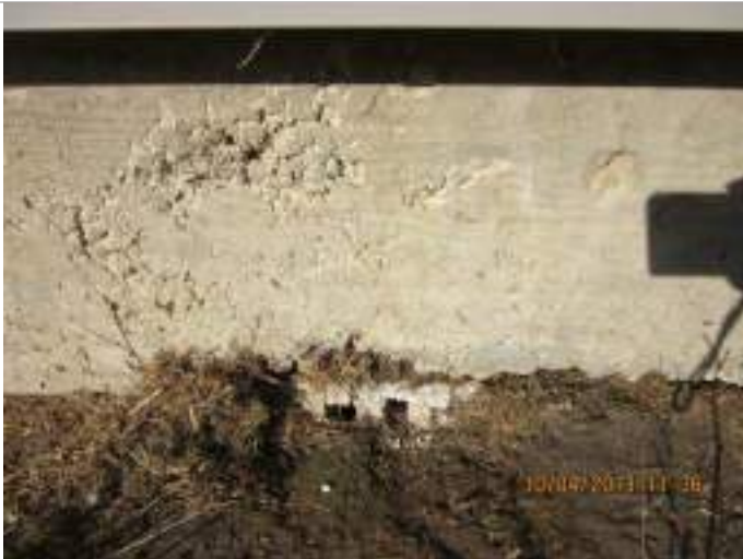
Photo 1: East side of building with voids and segregation of concrete foundation.
