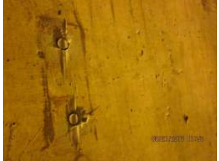
Photo 2: The wall of Dry Well has bolts that are cut off that need paint to prevent corrosion similar to these shown.
