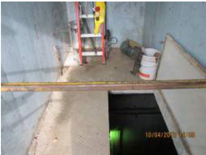
Photo 3: Cover the oversized pipe opening to prevent things falling into the Wet Well.
