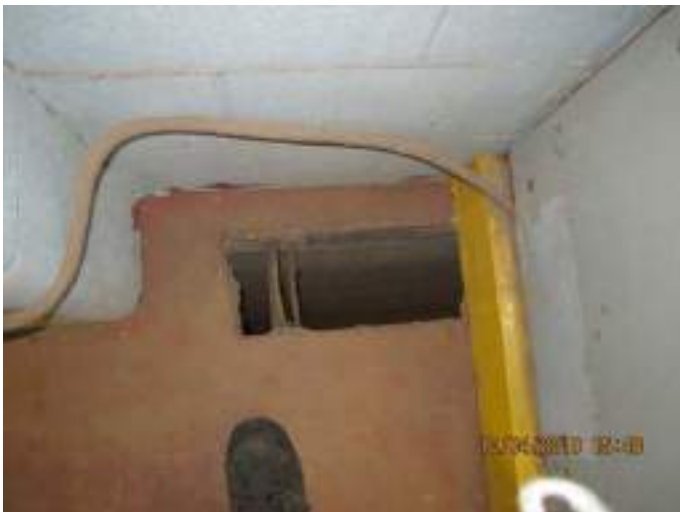
Photo 11: Opening in the main floor slab of the Dry Well where things can fall through into the Dry Well.
