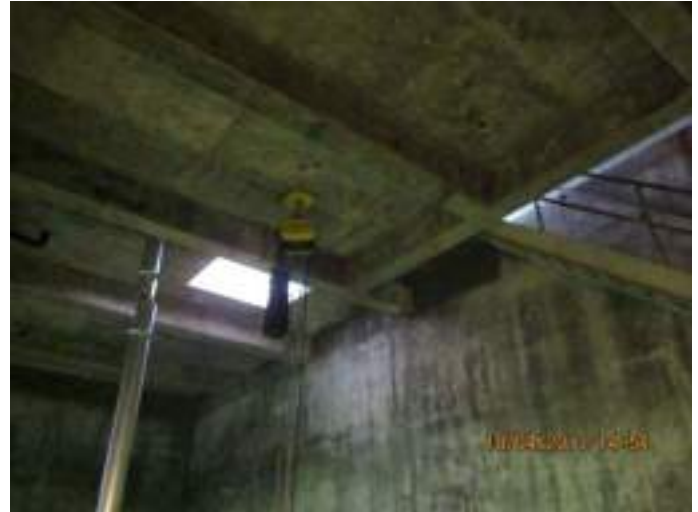
Photo 2: Hoist in Wet Well mounted to underside of main floor slab was being used to service equipment. The rated capacity and inspection sticker are not visible.
