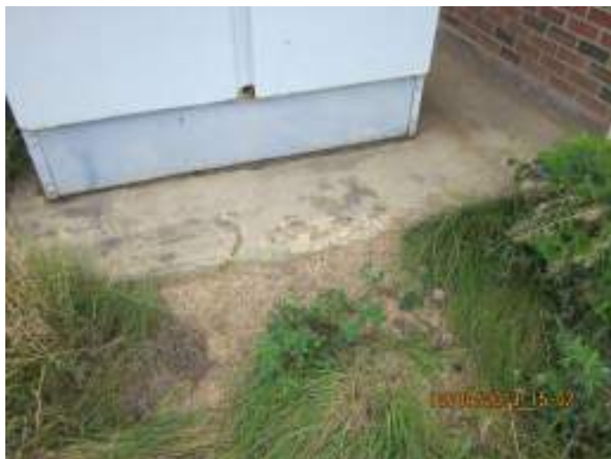
Photo 15: Concrete is spalling off a cabinet foundation on the north side of the building.
