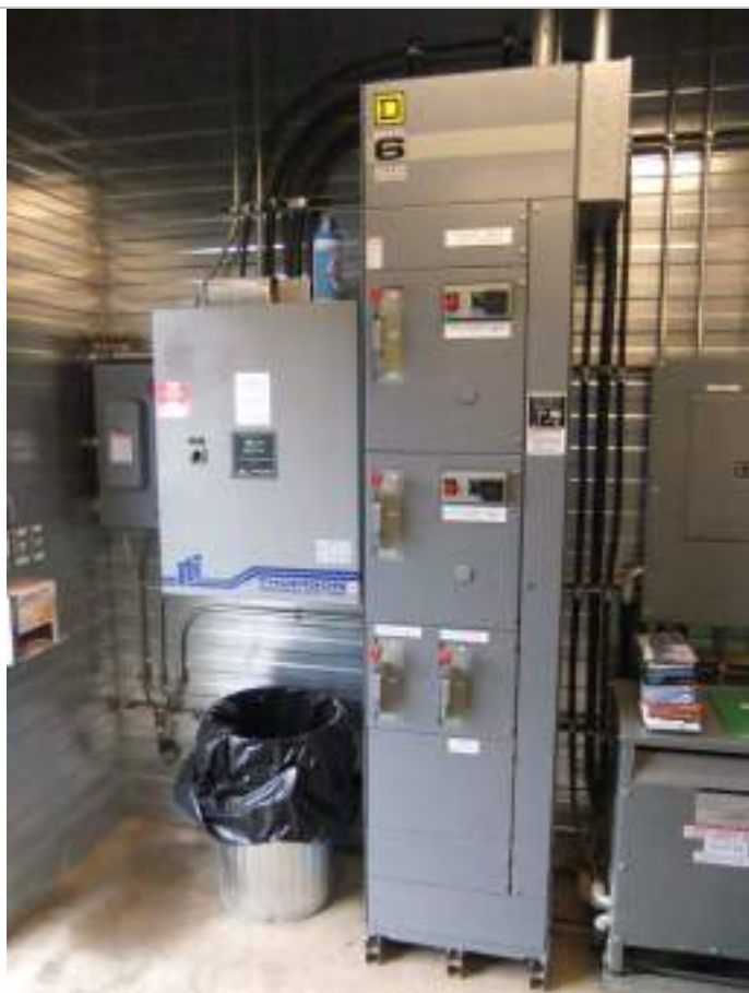
Photo 3: Transfer switch and MCC in good condition.
