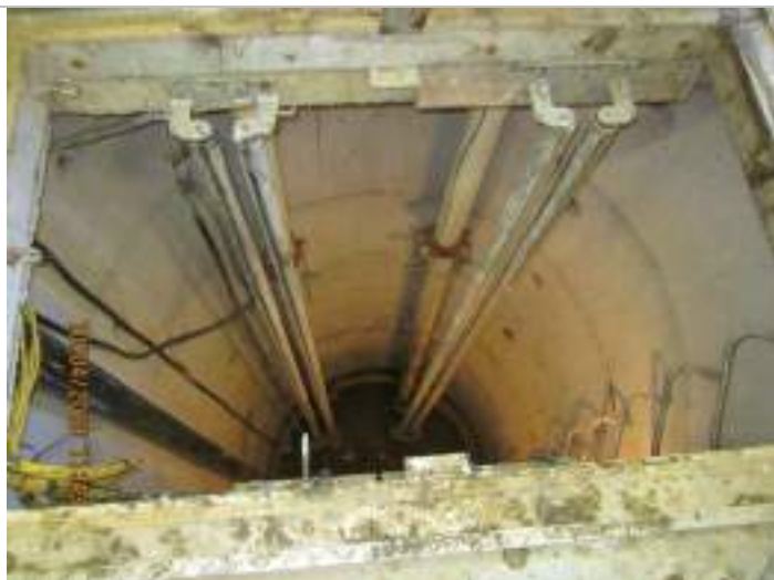
Photo 1: Discharge valves piping, above wet well access.
