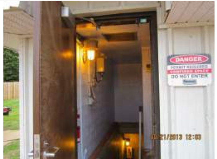
Photo 2: The pressure balancing is 'off' (notice dust trail along door and vent is fill with dust below).
