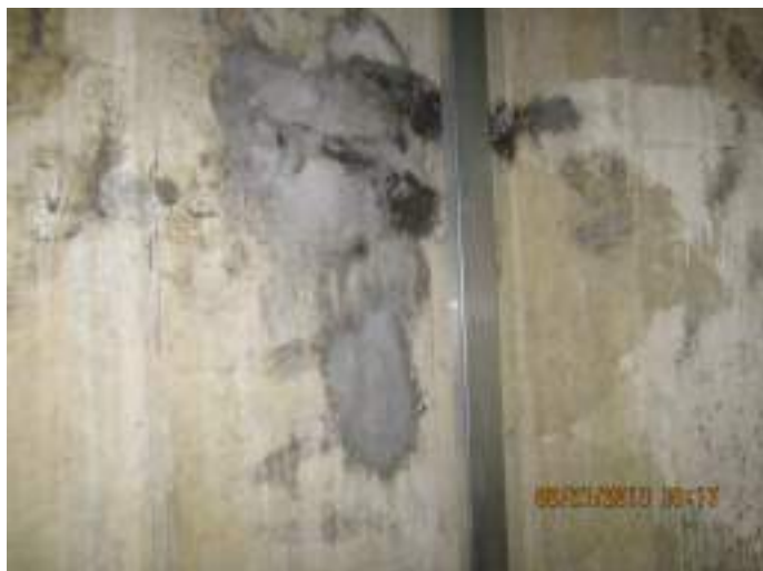
Photo 1: Dry Well concrete wall patch has minor cracking.
