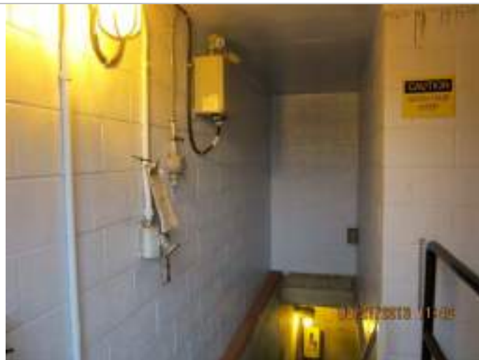
Photo 10: Masonry block wall in Wet Well stairway in good condition.
