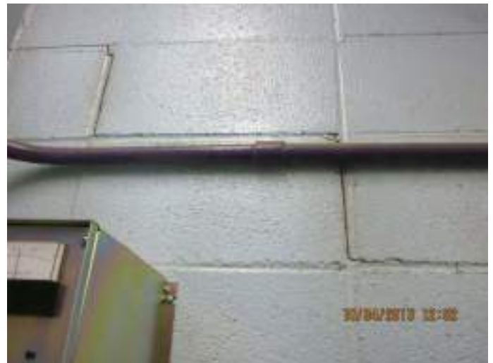
Photo 8: Cracks in joints of masonry block wall in Dry Well.
