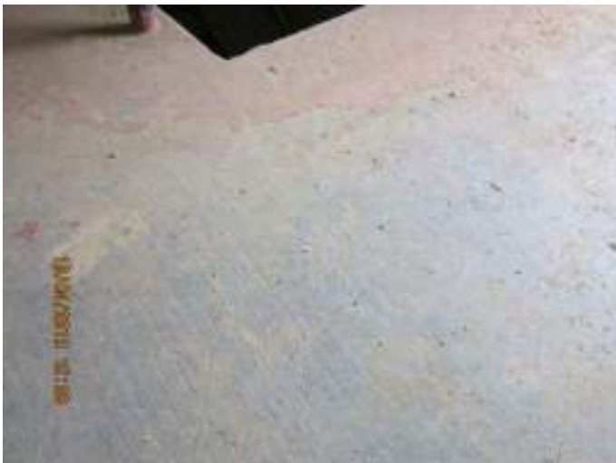
Photo 7: Shrinkage cracks in the Dry Well main floor slab near the stair opening.
