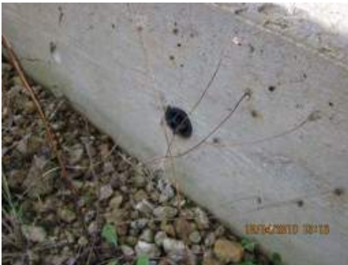
Photo 7: Remove form tie former and patch at antennae foundation.
