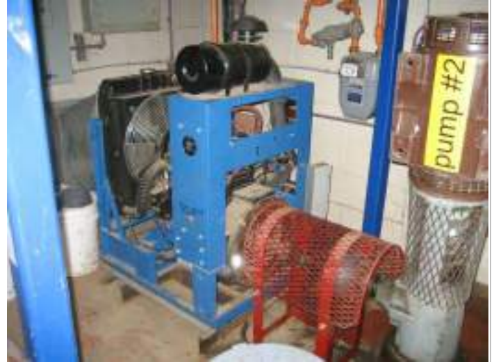
Photo 2: Pump #2 – motor & engine drives.
