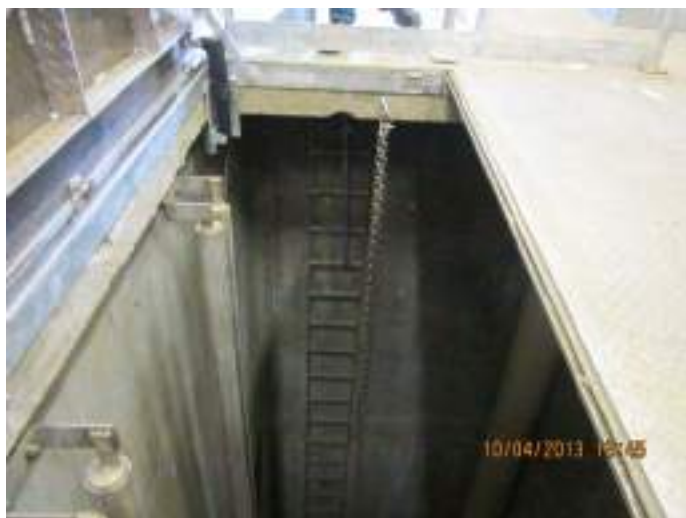
Photo 15: Access ladder down into the Wet Well with no safety cage. Fall protection is needed to enter on the ladder.
