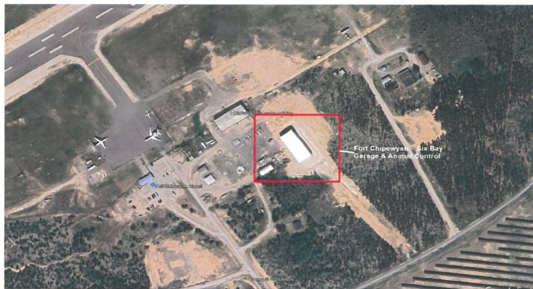
Aerial view of construction area.
