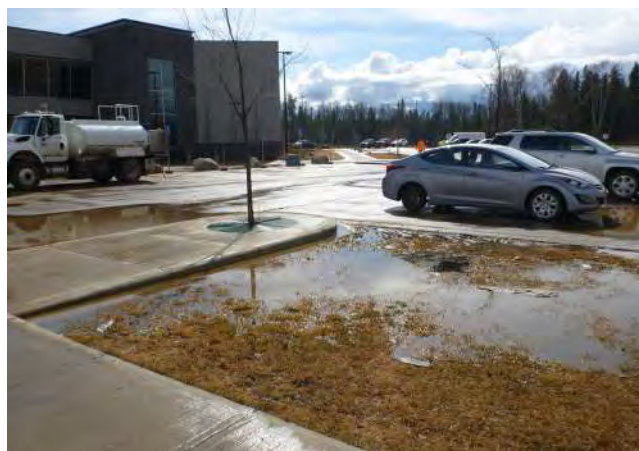
Improving FAC inspection procedures and recourse on latent defects would help to reduce maintenance by identifying deficiencies such as these drainage issues at the newly built Anzac Recreation Centre parking lot.
