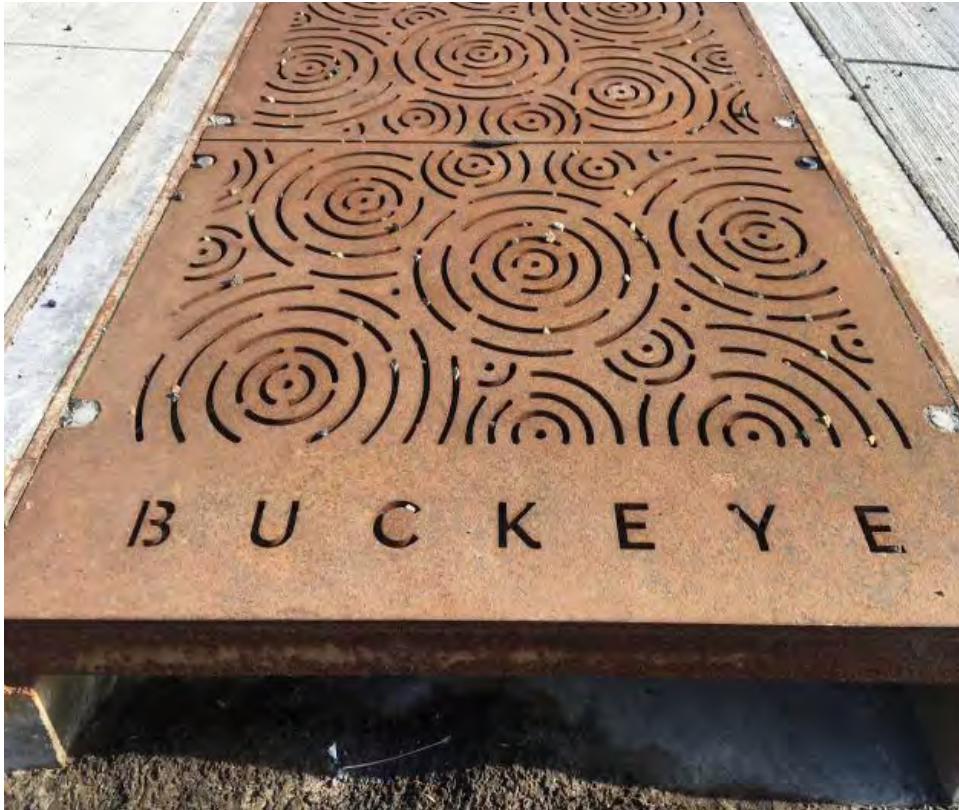
Stephen Manka, Cleveland, OH, USA: Iron grates: Part of a green infrastructure project, these grates were designed to decrease the amount of combined sewer overflows into the environment and eliminate neighbourhood sewers from being overwhelmed during big storms.
