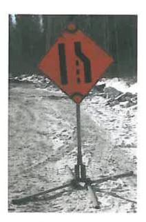
A-frame supports for warning signs are to be used ONLY for short duration use, lasting less than eight (8) hours e.g. "Men at Work" signs which are removed overnight, or for other "moving" operations.
