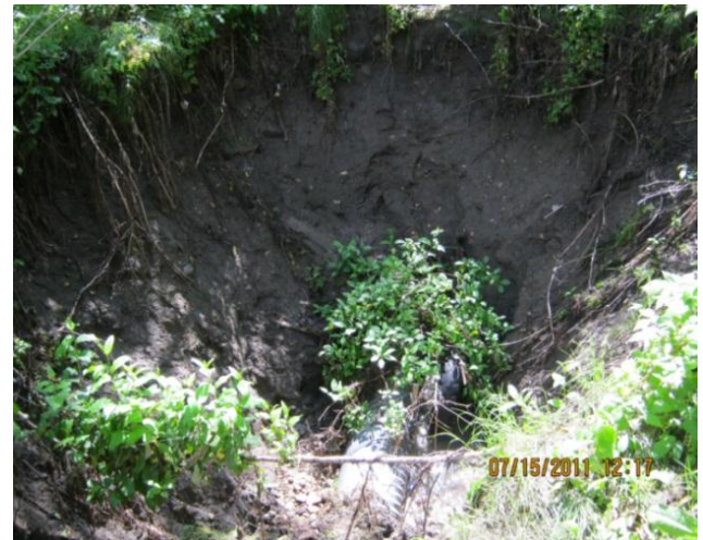
Sinkhole at base of slope on Beacon Hill storm sewer outfall line
