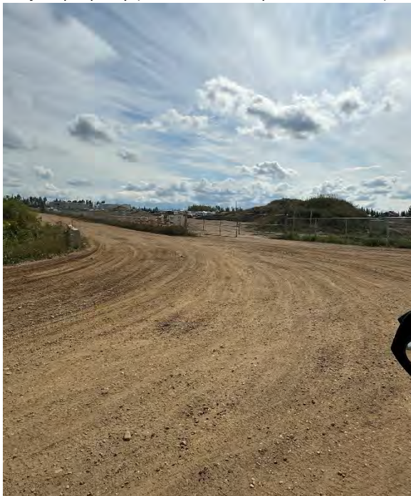
Photo 2: Southwards left entrance into subject property (4500 & 4520 Sapræ Creek Trail).
