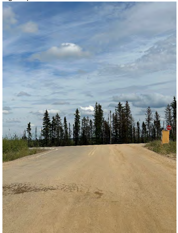
Photo 12: Road allowance towards Highway 69 (Saprae Creek Trail) with stop sign on the right.
