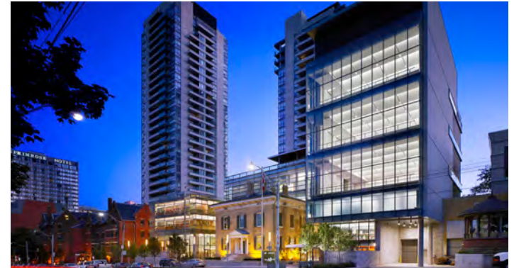
Example of lighting at the ground level
