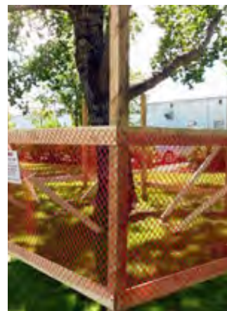
Example of tree protection during construction
