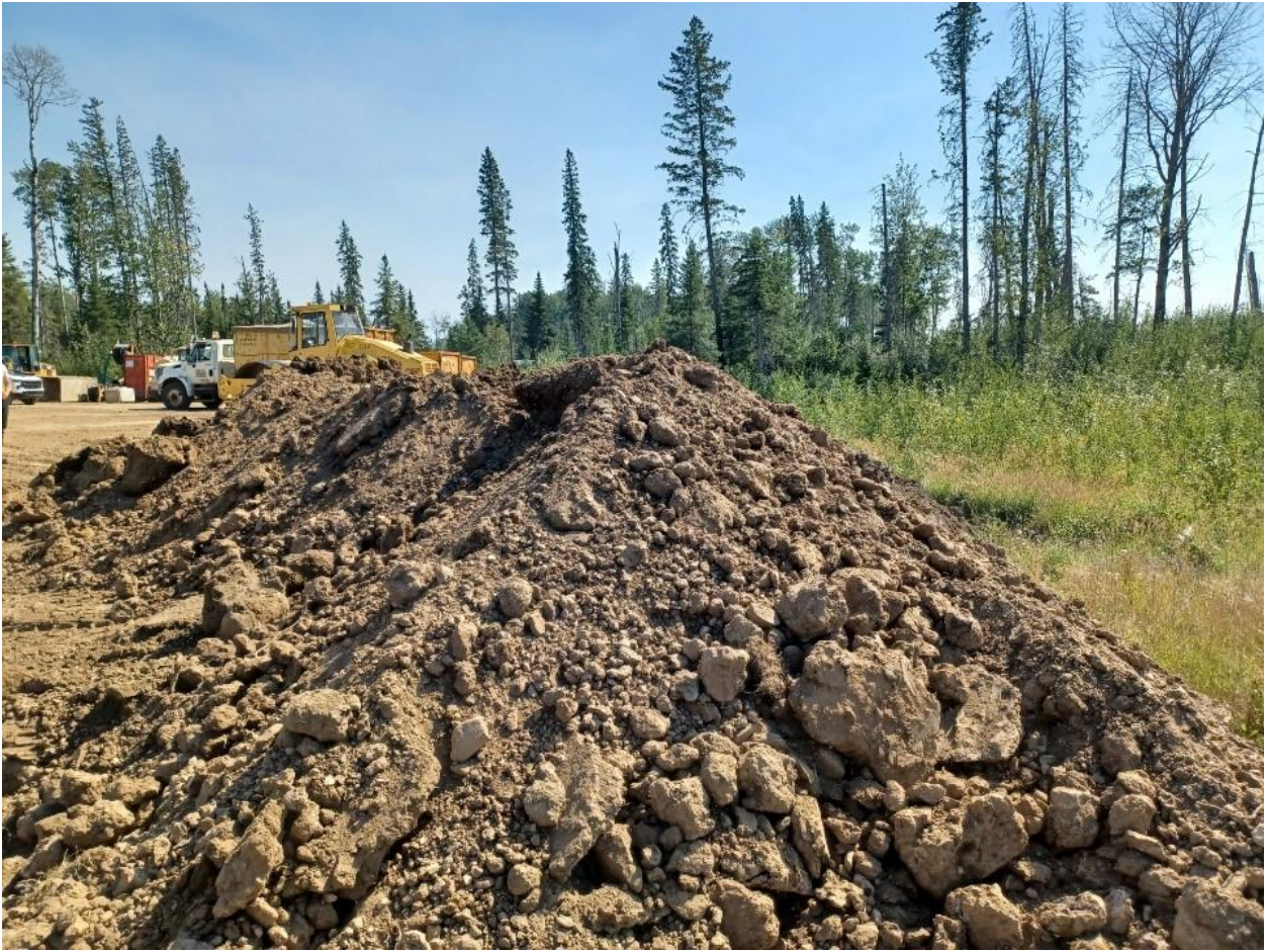
6. Excavation and Grading Alterations, Heavy Equipment, Commercial Vehicles
