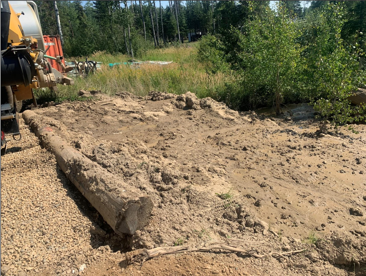
Photo 02: Hydrovac Waste Materials at the Site
