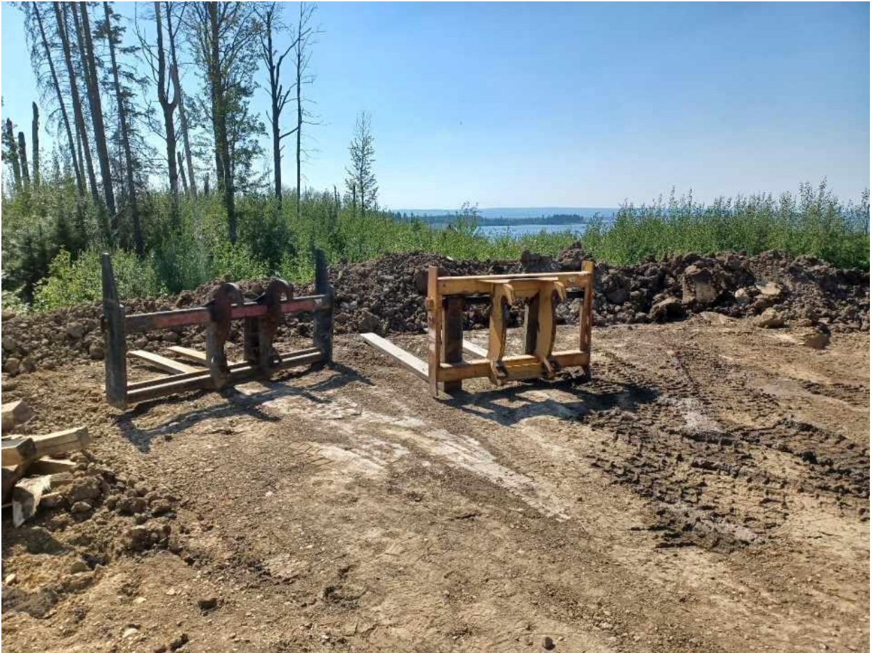
15. Heavy Equipment and Grading Alterations
