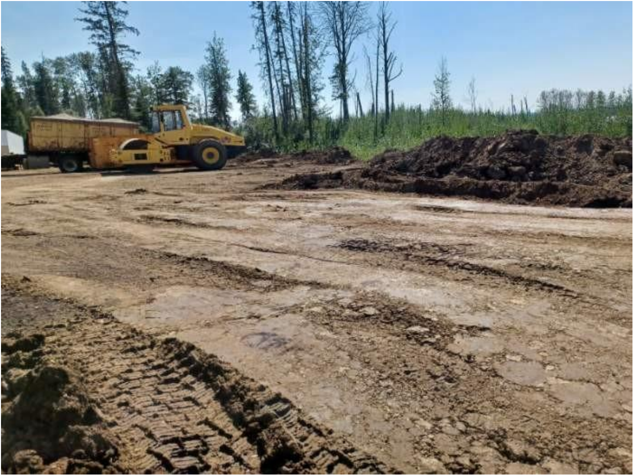
7. Excavation and Grading Alterations, Heavy Equipment, Commercial Vehicles
