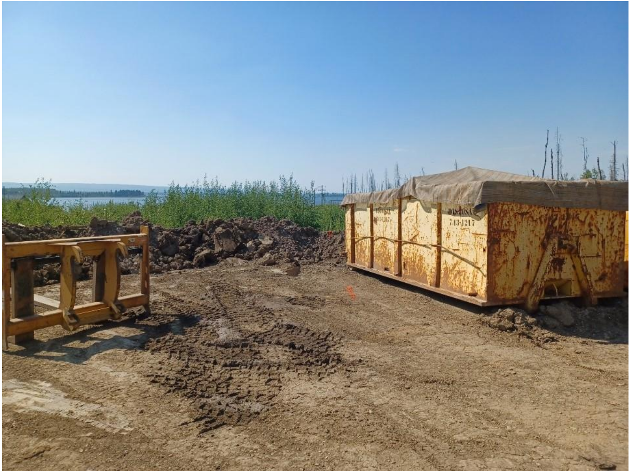
16. Heavy Equipment, Storage and Grading Alterations
