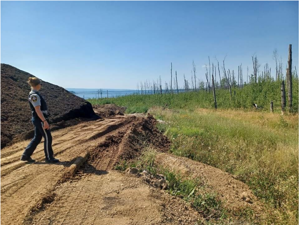
9. Stockpiling, Excavation and Grading Alterations
