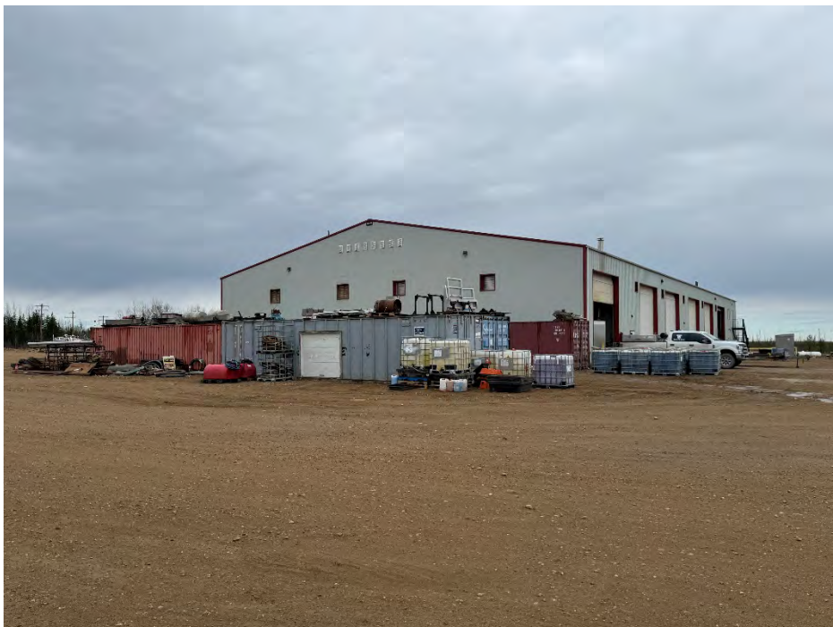
Pic 14 Rear and side view of the main building showing multiple container units, chemical storage tanks, and industrial materials placed along the wall
