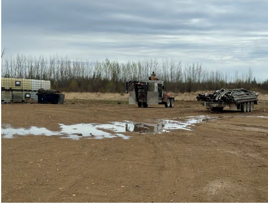
Pic 19 Pipes loaded on flatbed trailer and several IBC totes visible near the rear property boundary.
