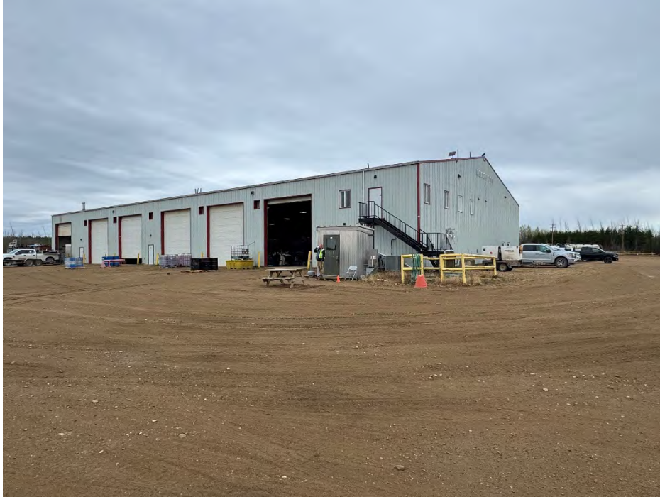
Pic 21 Main building with multiple bay doors open
