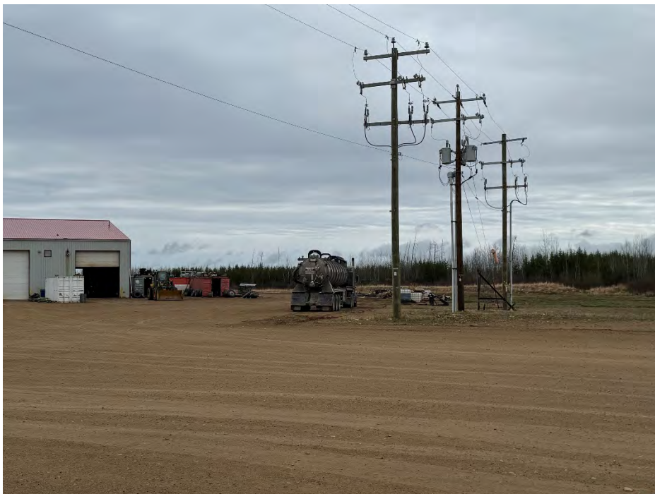
Pic 6 Rear area of the industrial building showing equipment, storage tanks, a hydrovac truck
