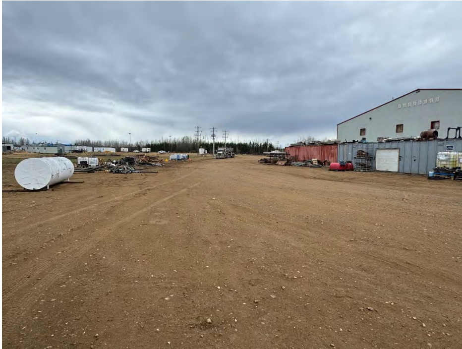
Pic 15 Wide view showing scattered industrial materials, large storage tanks, and containers adjacent to the main building
