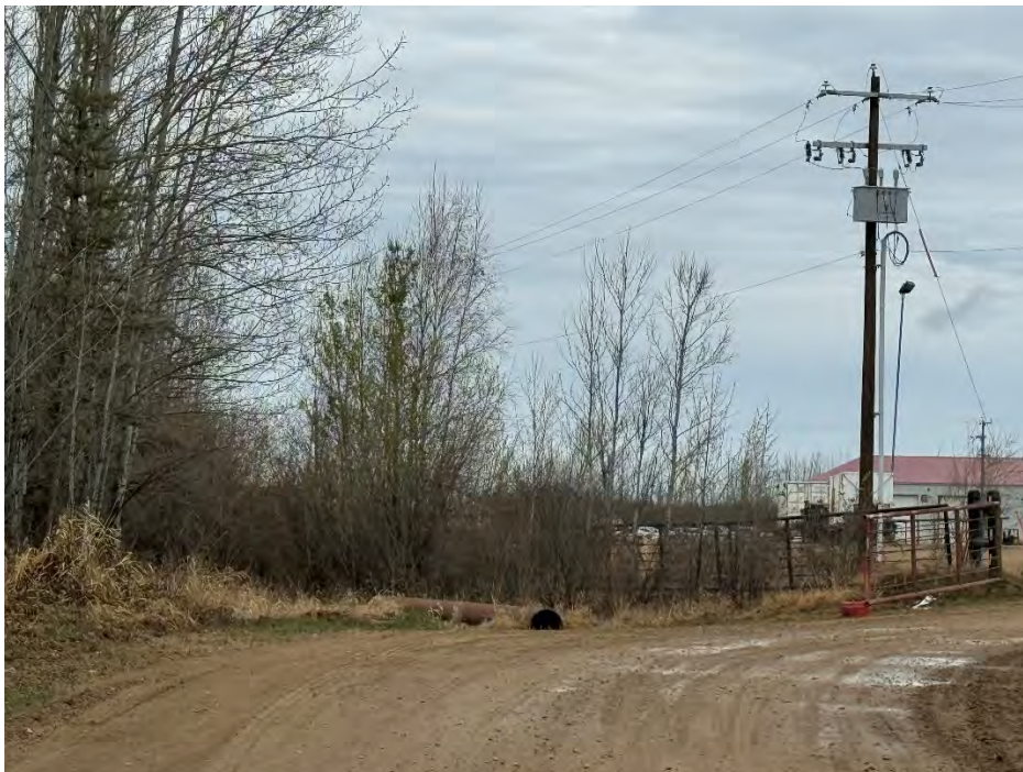
Pic 4 View of the site entrance from the access road
