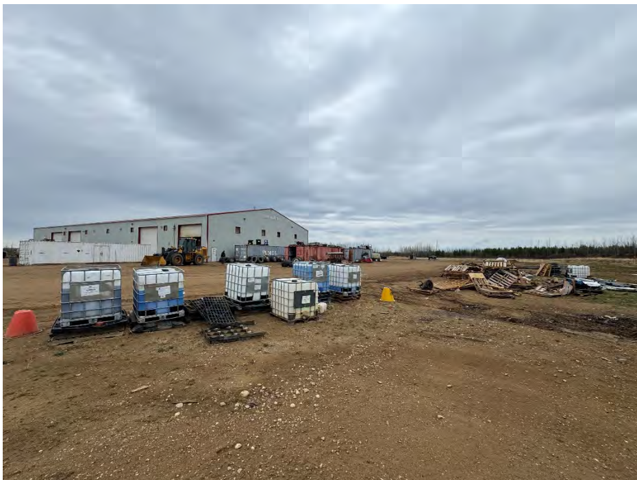
Pic 12 View of chemical containers, pallets, and scattered equipment placed on open ground
