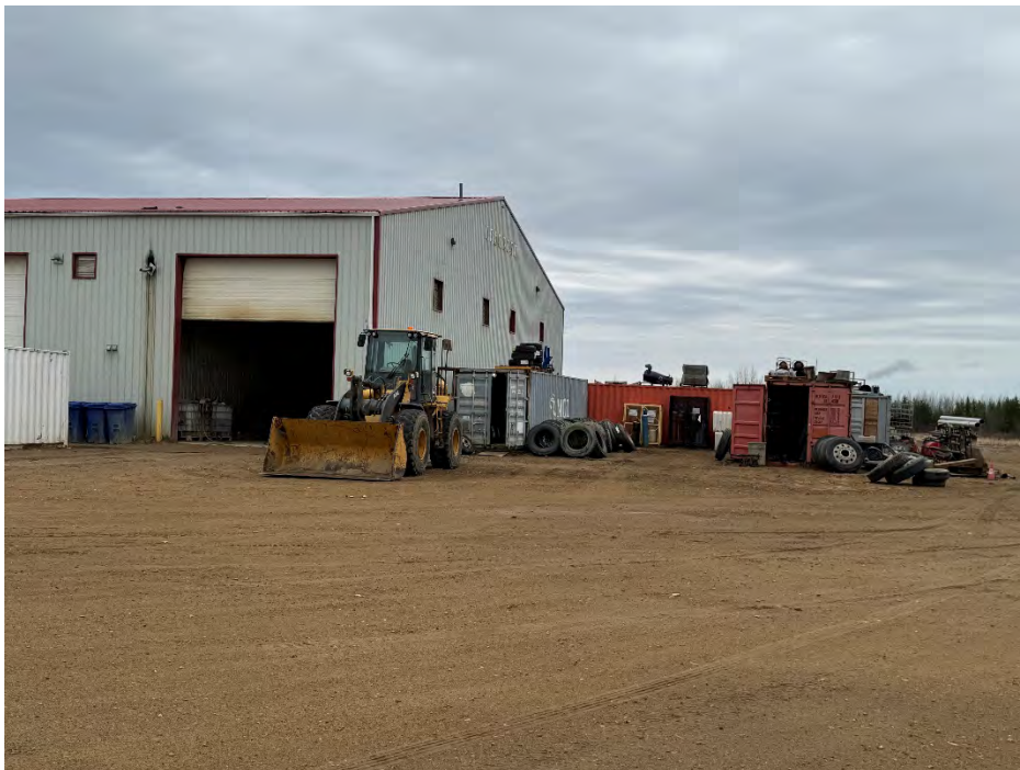
Pic 10 Equipment and material storage beside the building, including tires, containers, and machinery
