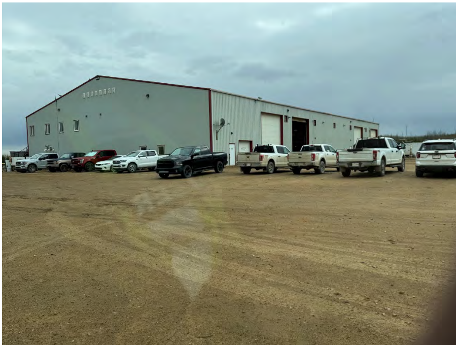
Pic 36 North-South view of the main industrial building with multiple service bays open and several employee and service vehicles parked along the façade.
