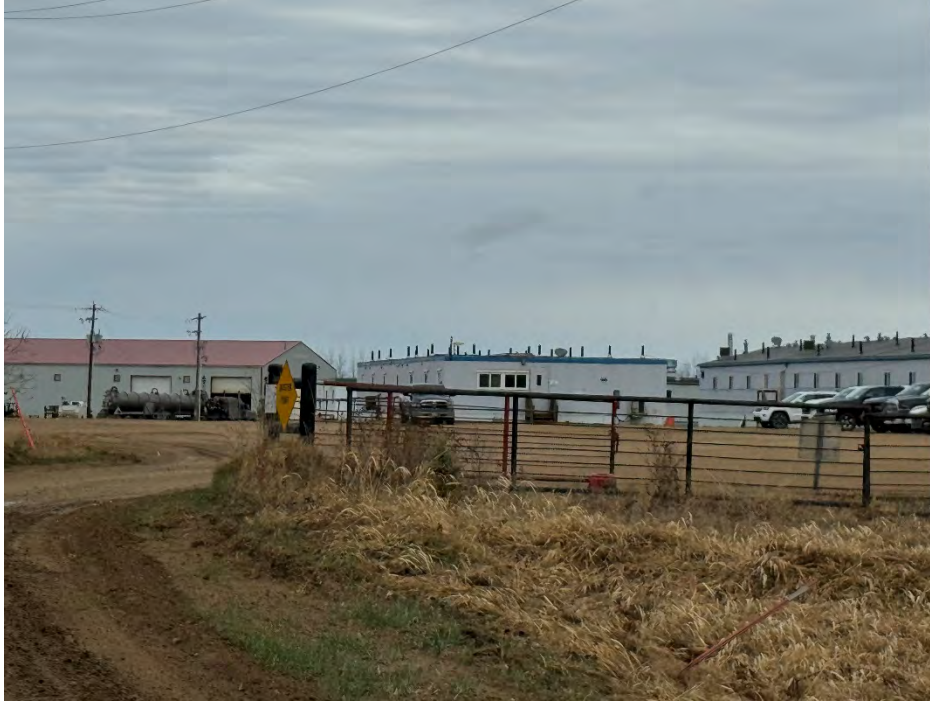
Pic 3 View of the main building with open bay doors and industrial equipment visible, along with camp structures and multiple parked vehicles.
