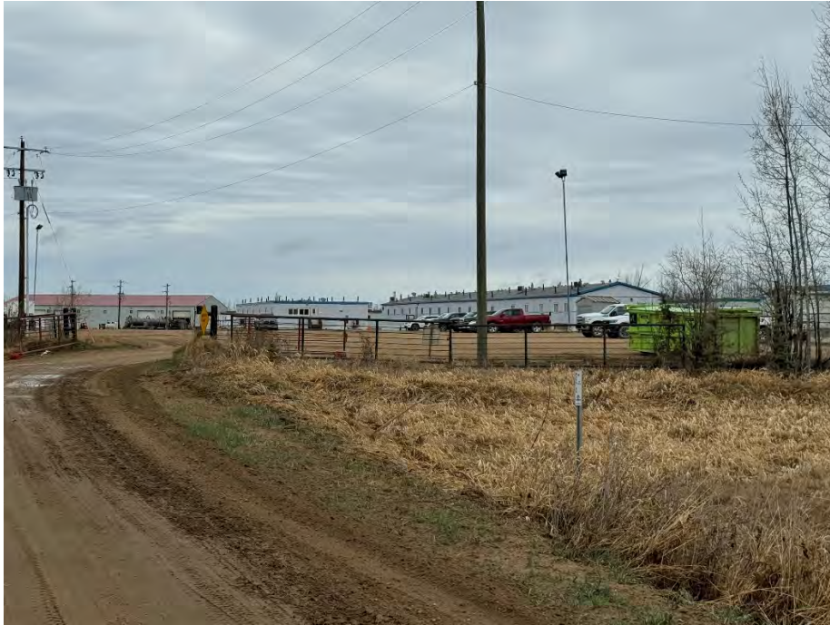
Pic 1 Entrance view showing multiple buildings, parked vehicles, and site fencing with a security gate.
