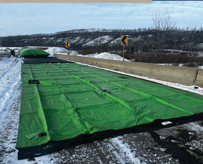
Installation of triple dams adjacent to Clearwater Drive in preparation for river breakup.
