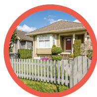
Combustible Wooden Slat Fence
